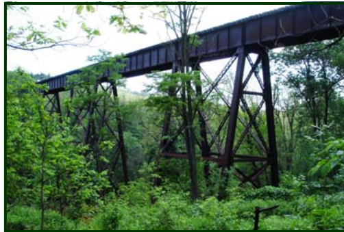
Viaduct Bridge –Snow Shoe Rail Trail
