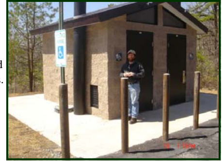
Restroom Facility at Gillentown Trailhead
